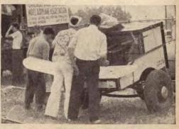
A simple "box" type trailer of small size will conveniently serve smaller model clubs. This one was built of scrap lumber and mounted on a junk yard wheel and axle assembly.
